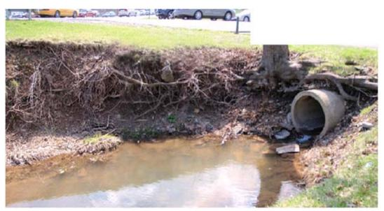
Figure 3-15 Erosion of Miller Run stream banks on the west side of Route 15
